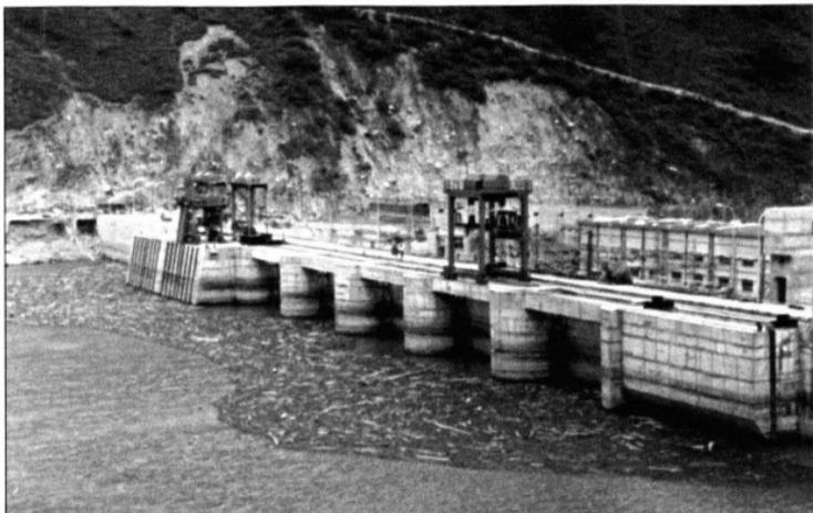
*Accumulation of debris upstream near fish exit*
